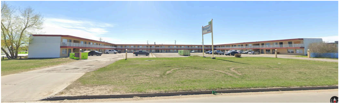
Photo 1 — Existing building at 11301 100 Avenue, set back approximately 6 metres from the service road.
