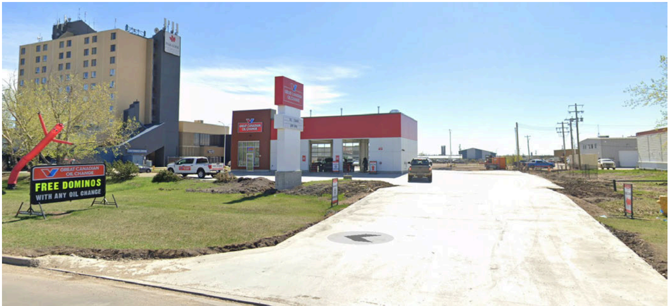
Photo 5 — Frontage at 11251 100 Avenue: pylon sign, fascia signage and open service bays.
