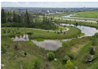
Storm Infrastructure Upgrades and Replacement
