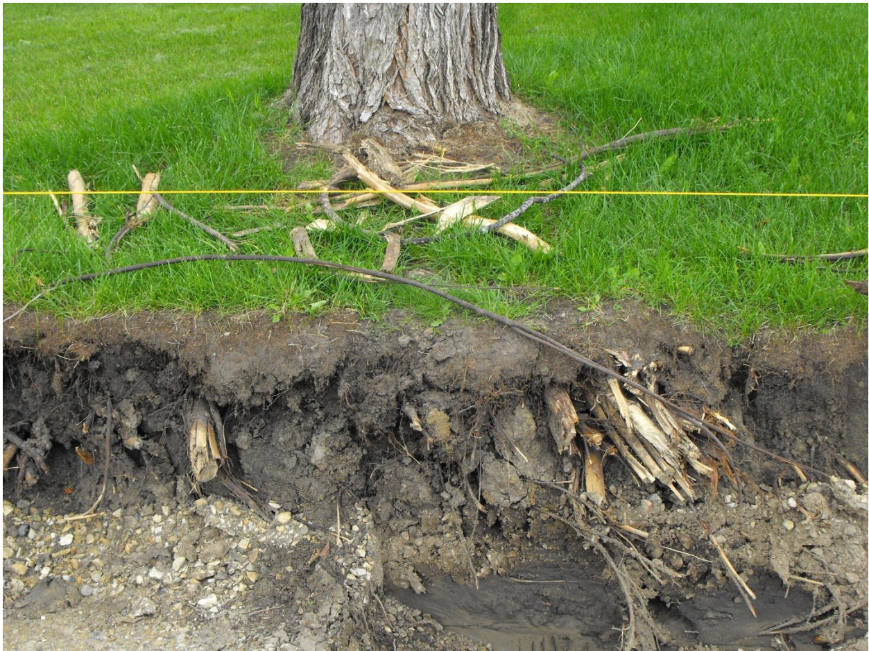
Sidewalk replacement excavation
